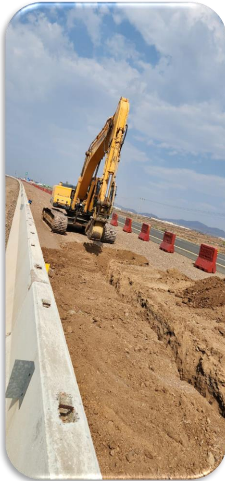
Excavation work for OFC laying
